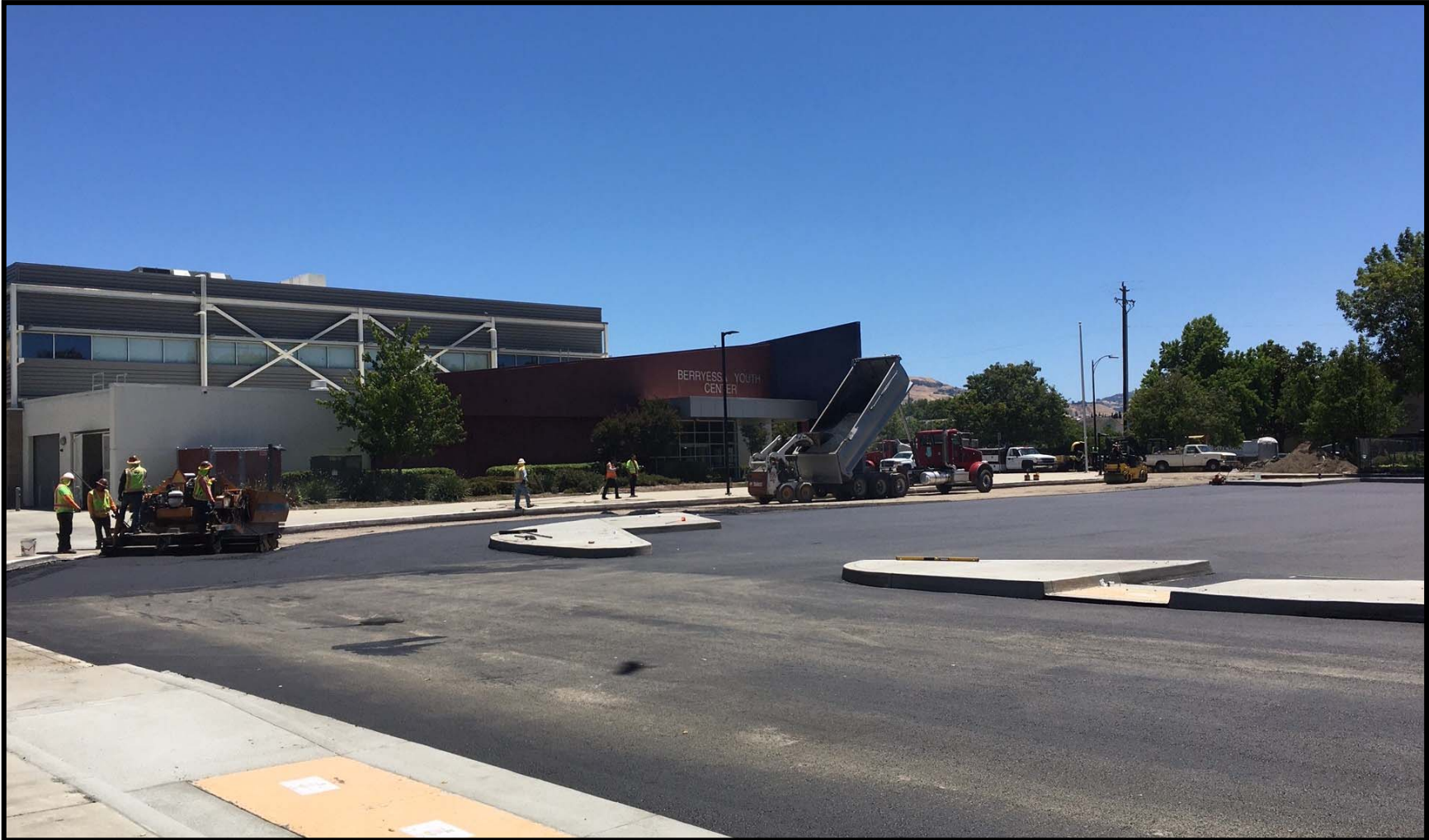
Morrill Parking Lot
