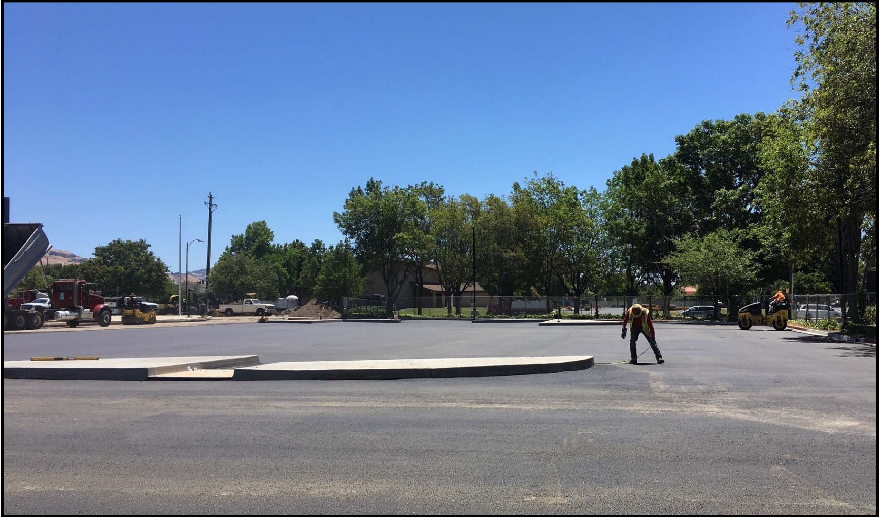
Morrill Parking Lot
